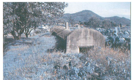
移設前の掩体壕
